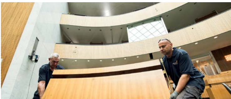
Furnishings of the plenary hall of Parliament building being dismantled
